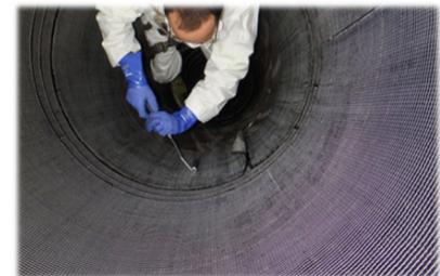
Self-adhesive SAERfix carbon non-crimp fabrics from Saertex were used in this case. These tacky fabrics helped the workers for the lay-up, especially in the vertical sections of the existing pipe.
